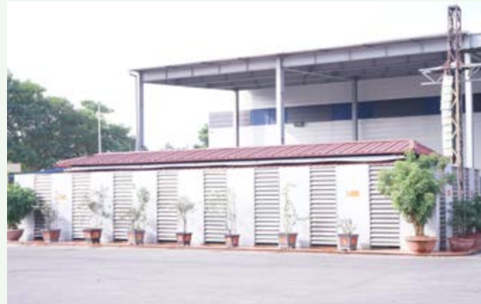
▲ Bồn ngầm Cyclopentane 35m 3 / Cyclopentane Underground 35m 3 Storage Tank
